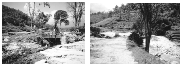
Fig.1 The flood and landslide event at Mae Rak sub-watershed, Ping river basin. (September,16,2002)
